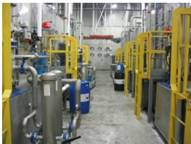
The line prepares the rim's alloy metal surface for liquid and powder painting using a 15 stage pre-treatment system, supported by 10 chemical dosing, mixing and storage vessels, all with their own pumping, flow and temperature control systems.
